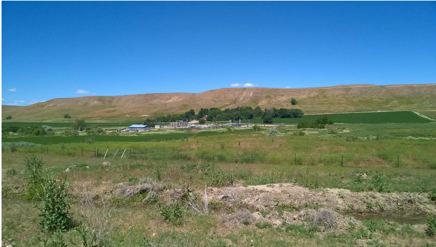
LITTLE WILLOW GATHERING FACILITY PAYETTE CO. ID LOOKING SW FROM ML 2-10 WELL PAD, JUNE 2017 PHOTO COURTESY J. THUM
