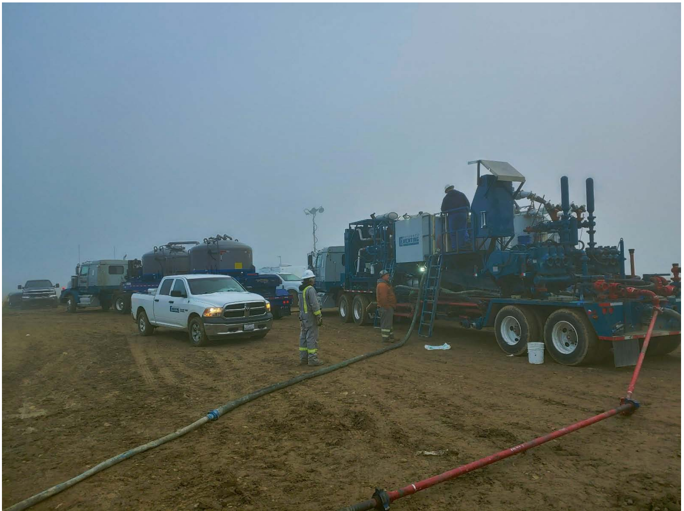
Resource Cementing equipment and crews set up for surface casing cement.
