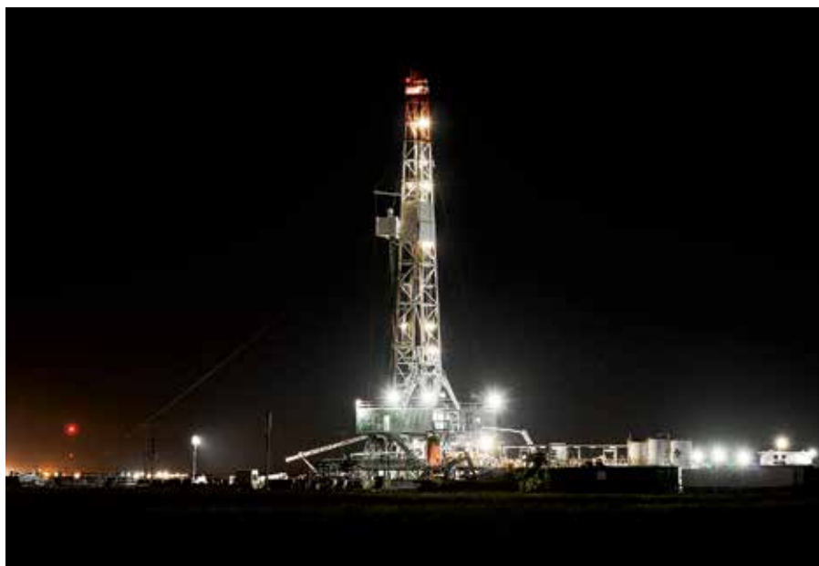
Fig. 1. As of September, U.S. rig activity was down 76% from Jan. 4, 2019, as exemplified by Ensign rig T223, drilling for Parsley Energy at Pecan State Unit 4303JH, as it targets the Lower Wolfcamp formation. The site is near the town of Coyoanosa, in Pecos County Texas. For another view of this site, please see this issue's front cover. Image: Parsley Energy.
