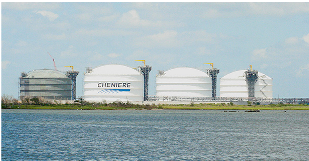
Cheniere Energy Inc.'s Sabine Pass liquefied natural gas terminal on the border between Texas and Louisiana. Roy Luck/Flickr
