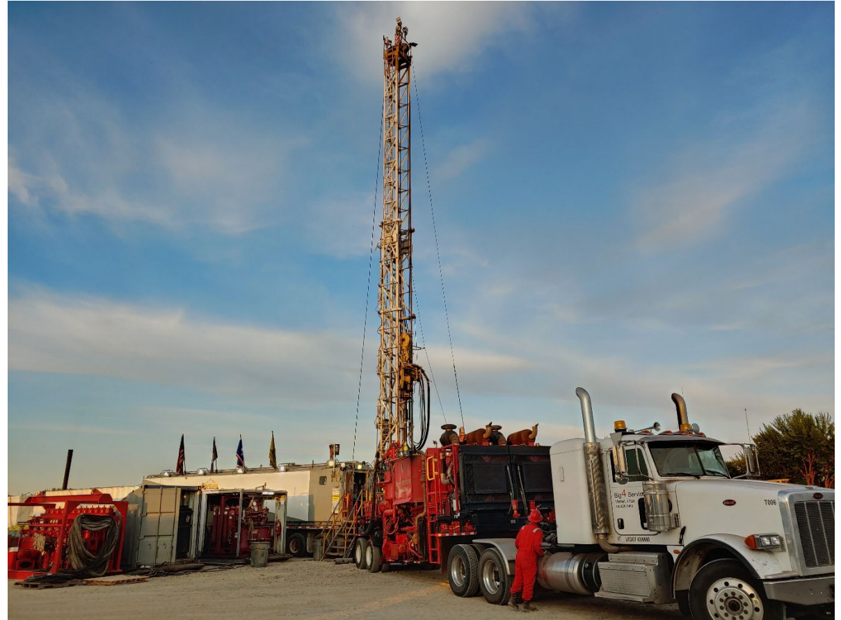
Surface casing cementing operations on the James #1-10, Payette County, June 2026. Photo courtesy J. Thum
