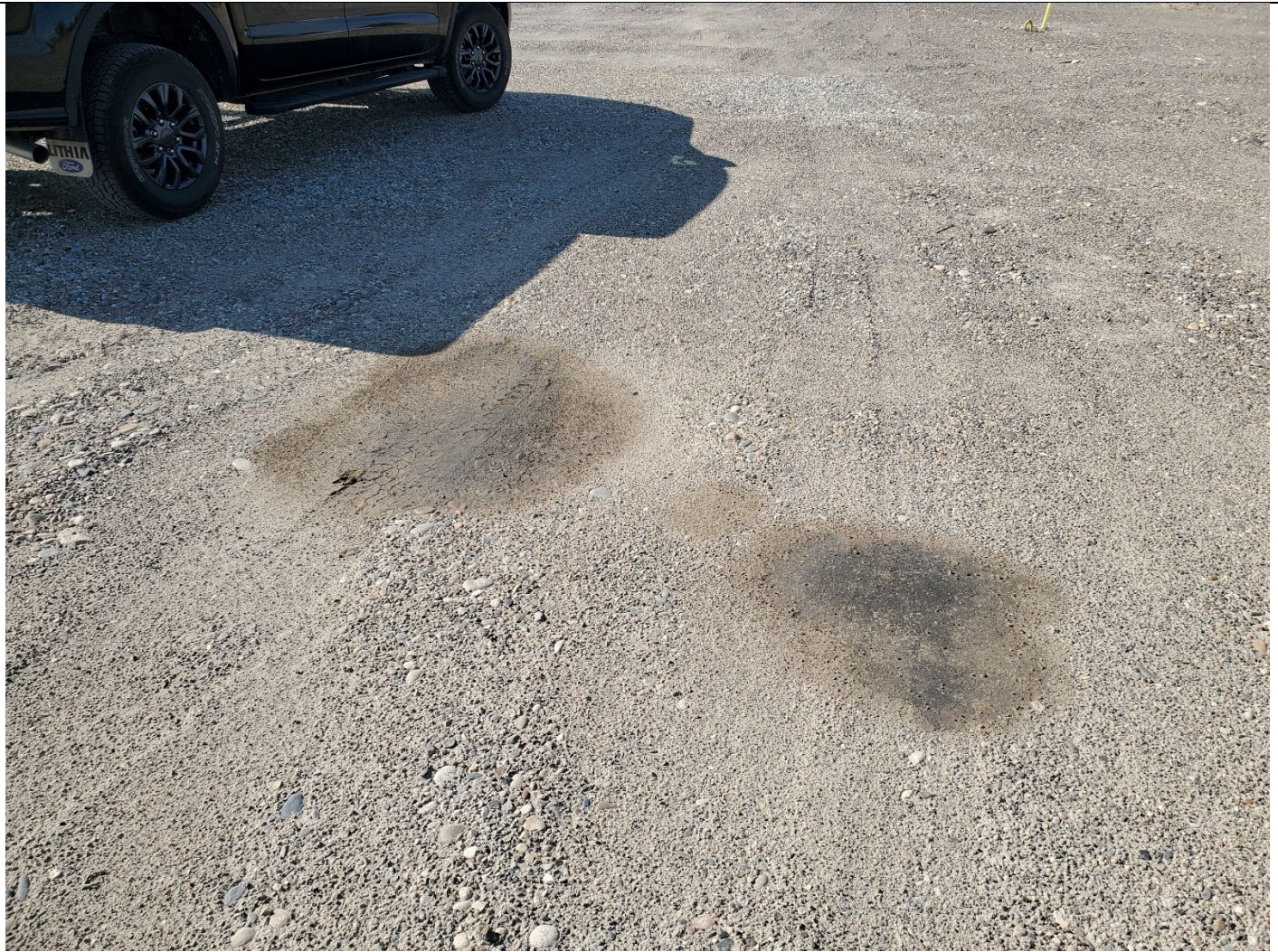
Hydraulic fluid stains, west side of pad.
