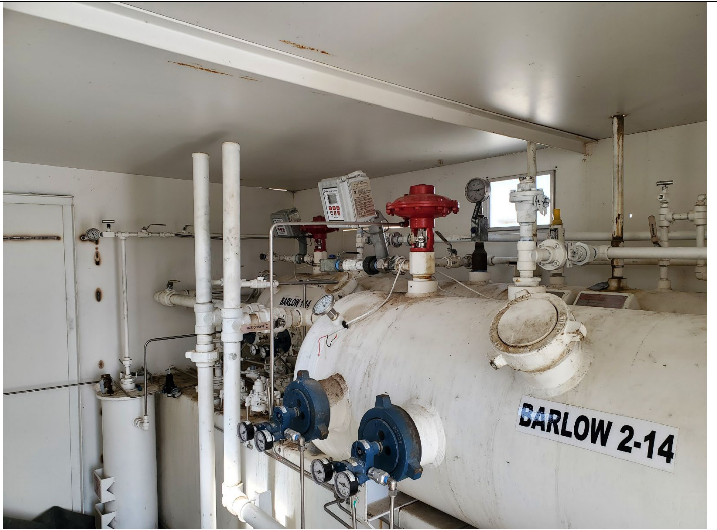
Barlow #1-14 and Barlow #2-14 double separator unit interior.
