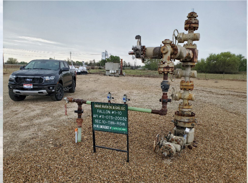
FALLON #1-10 ANNUAL WELL INSPECTION, APRIL 2024 PHOTO COURTESY J. THUM
