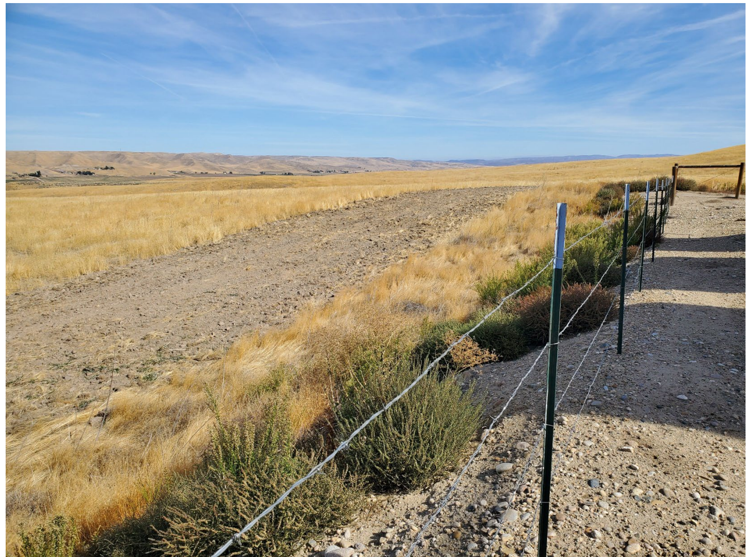
Bladed firebreak around pad for protection from August 2024 Paddock Fire. View is Northeast up Little Willow Canyon along north perimeter of the well pad.
