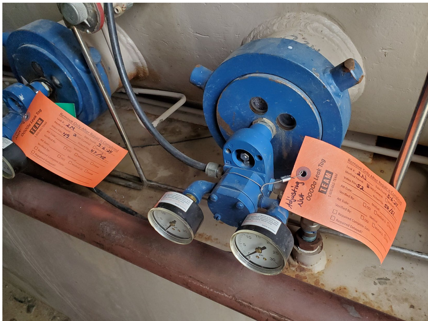
Photo 114902: Leak tags on pneumatic valves on separator, dated 3/6/2024. Operator is currently converting pneumatic valves to nitrogen-actuated systems for all wells and facilities to comply with 2024 EPA emissions requirements.
