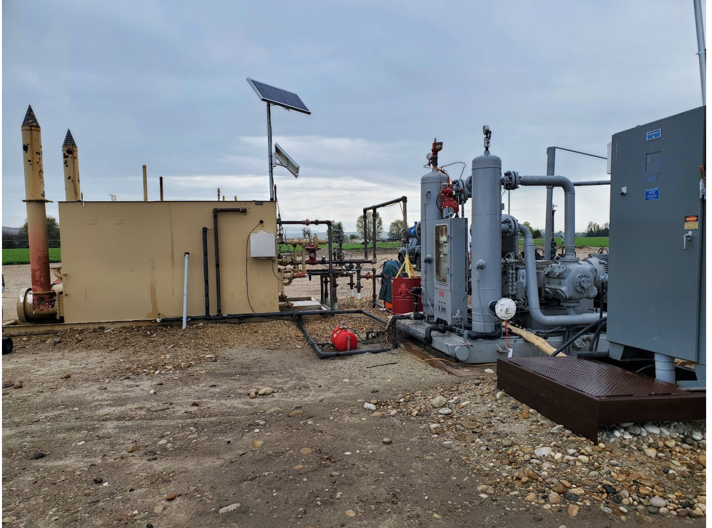
Photo 115120: Partial view of compressor unit on right, separator unit on left. View is east.
