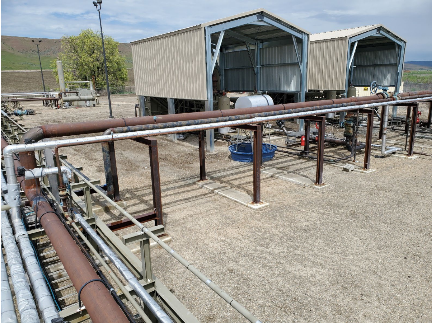
New compressor canopies, view North-Northwest
