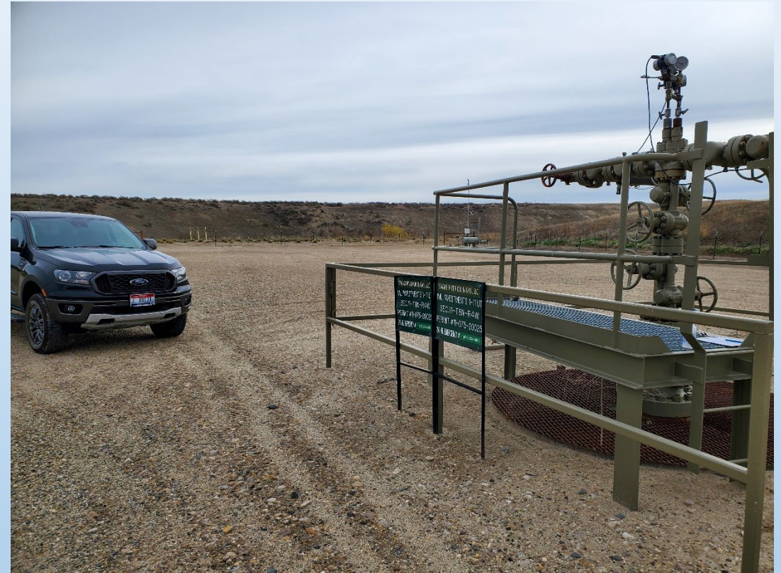
ML INVESTMENTS #1-11 WELLHEAD DURING ANNUAL INSPECTION NOVEMBER 2023 PHOTO COURTESY J. THUM
