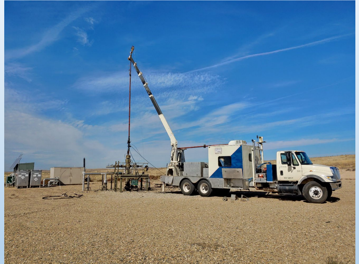
MODIFIED GAS LIFT OPERATIONS ON THE KAUFFMAN #1-9 WELL TO RE-ESTABLISH PRODUCTION, OCTOBER 2023 PHOTO COURTESY J. THUM
