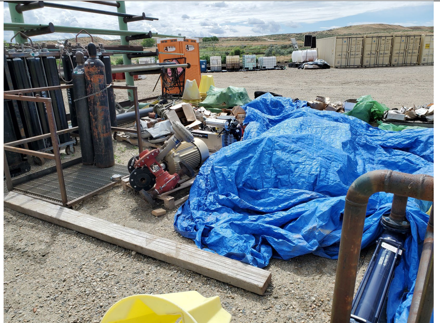
Temporary storage location of equipment and materials being utilized for current maintenance and installation operations. Stockpile is located in the northeast corner of the facility. View is south-southeast. Portable spill containment berm with palletized chemicals in background center.
