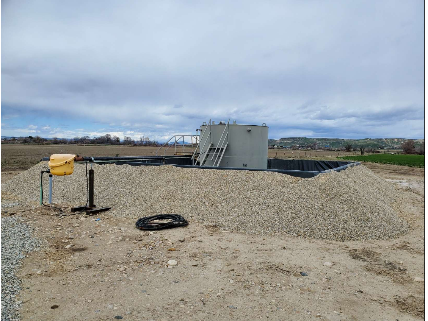
100-barrel capacity produced water tank and containment dike, north side of pad. View north 4/12/2023.
