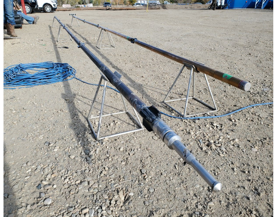
DIRECTIONAL DRILLING INSTRUMENTATION FOR THE BARLOW #3-14 OCTOBER 2022 INSPECTION TO WITNESS SURFACE CASING PHOTO COURTESY J. THUM
