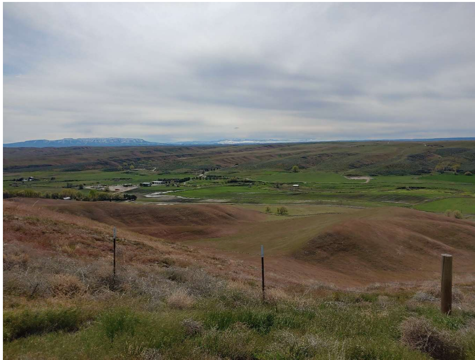
LOOKING SOUTHEAST TOWARDS LITTLE WILLOW GATHERING FACILITY AND THE EASTERN WELL PADS OF WILLOW FIELD, PAYETTE CO. ID. MAY 2022 PHOTO COURTESY J. THUM
