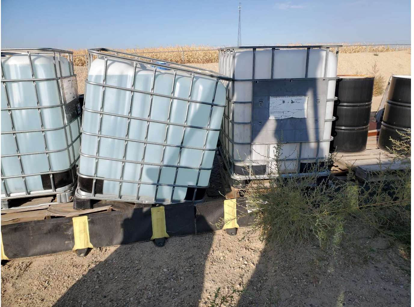
Broken pallet holding chemical tanks inside portable spill berm. NW side of facility, view West.
