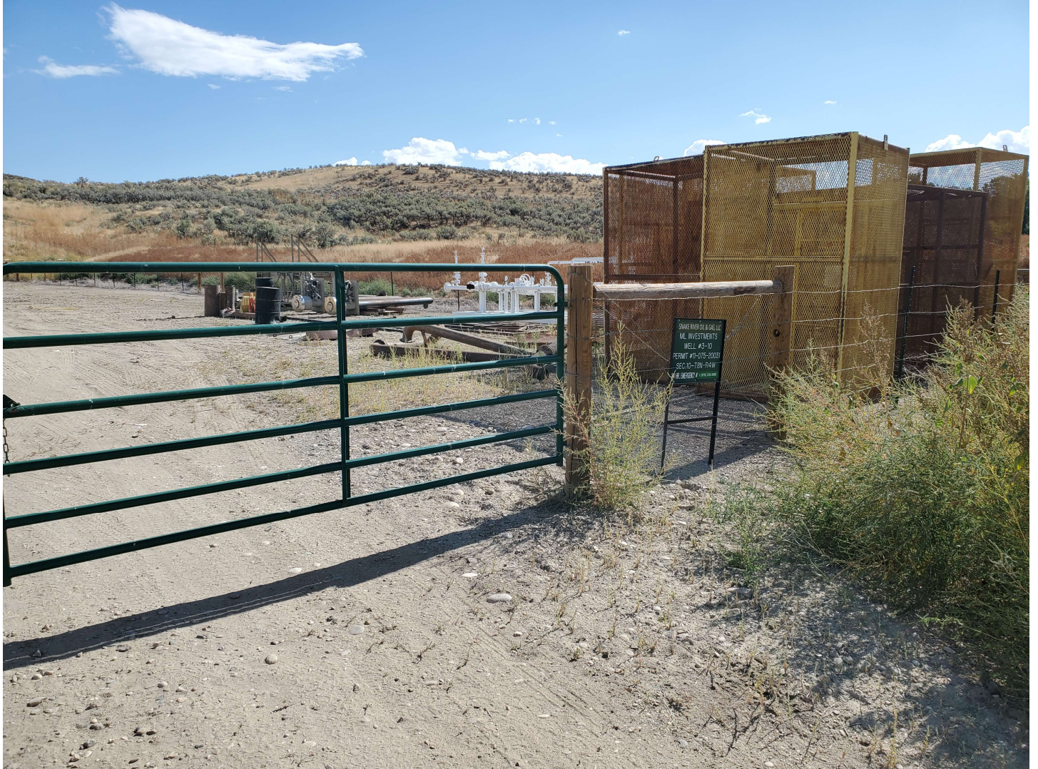
Entrance to well pad, view south. Spare equipment stored along SW fenceline.
