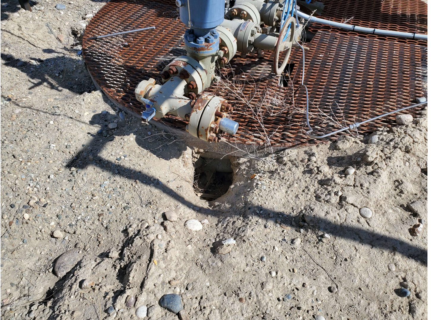
View of animal burrowing activity around cellar casing.
