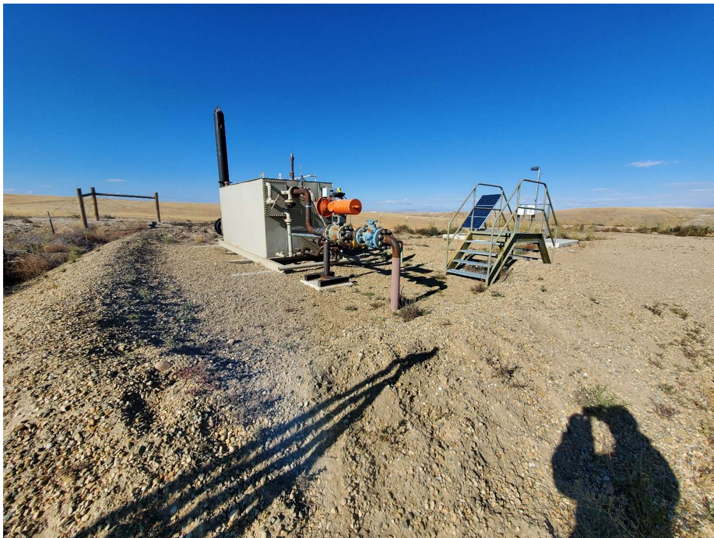
Separator unit and tank dike looking south. Note footprints of livestock traffic on and within containment dike.
