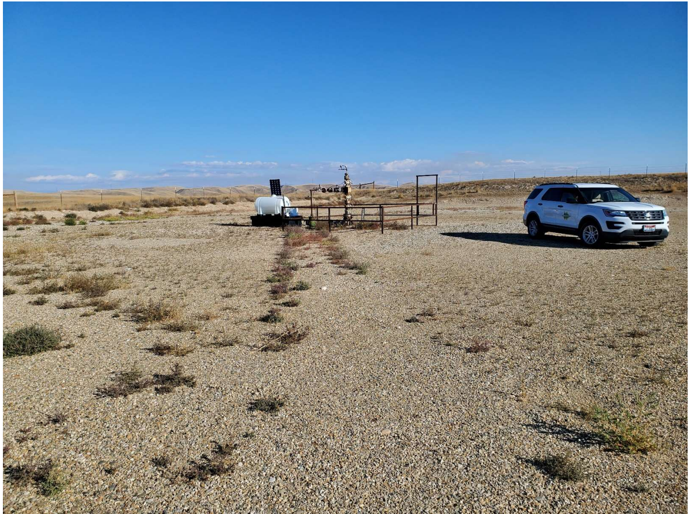
Well head and scavenger unit, looking north showing vegetation encroachment on well pad
