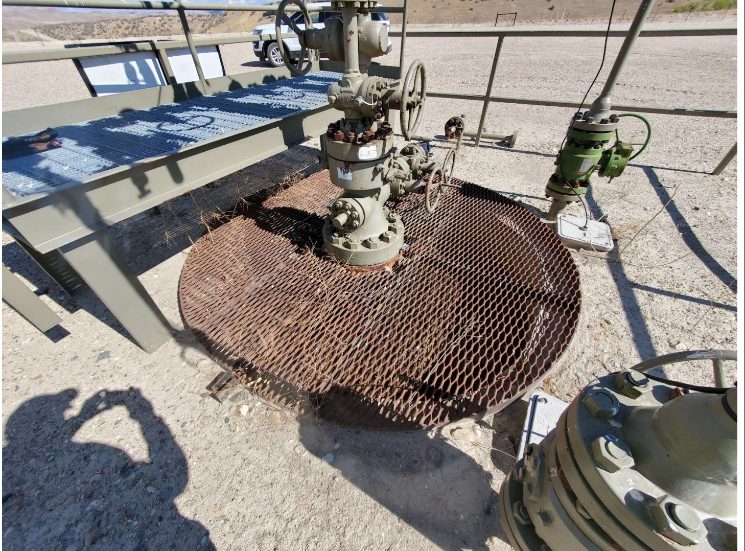
Cellar and protective cover.
