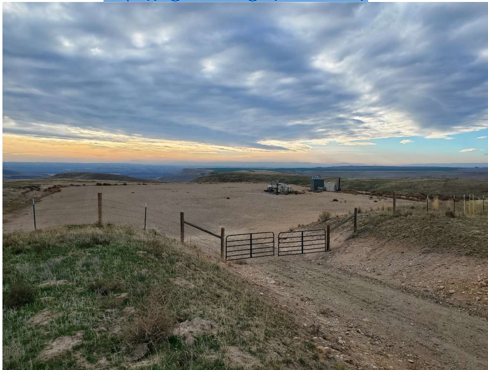
KAUFFMAN #1-9 WELL PAD LOOKING SW PAYETTE CO. ID NOVEMBER 2021 PHOTO COURTESY J. THUM
