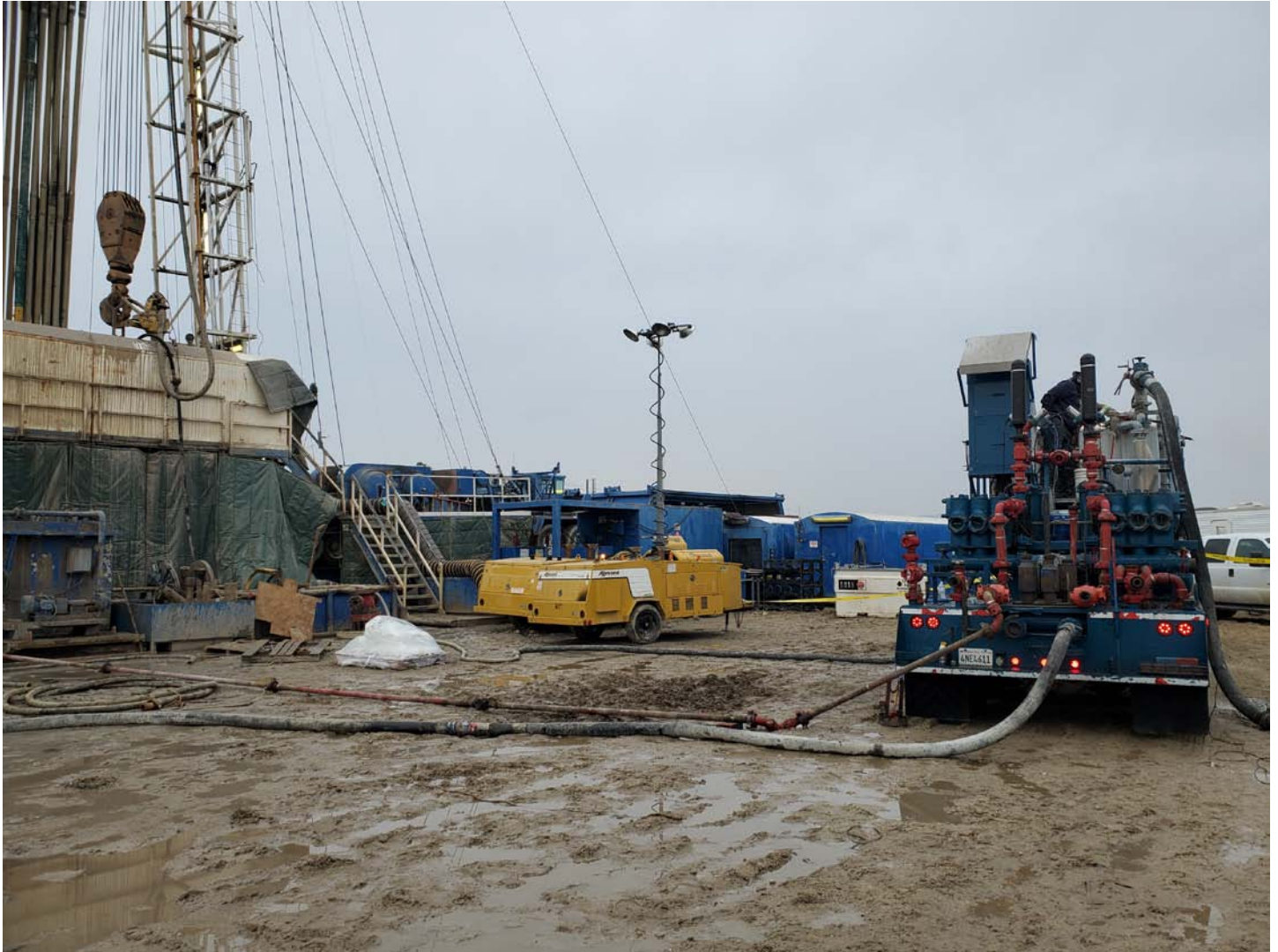
Resource Cementing equipment at start of surface casing cement job.
