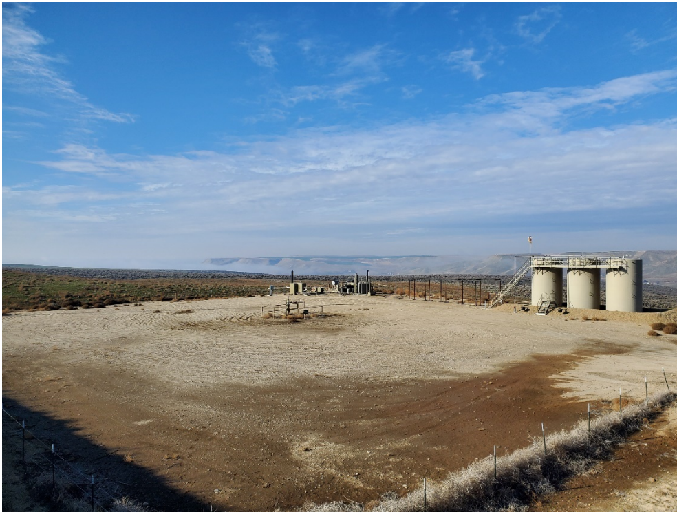
Overview of well pad looking WNW. Produced water tank batteries to right, wellhead center, separators back center.
