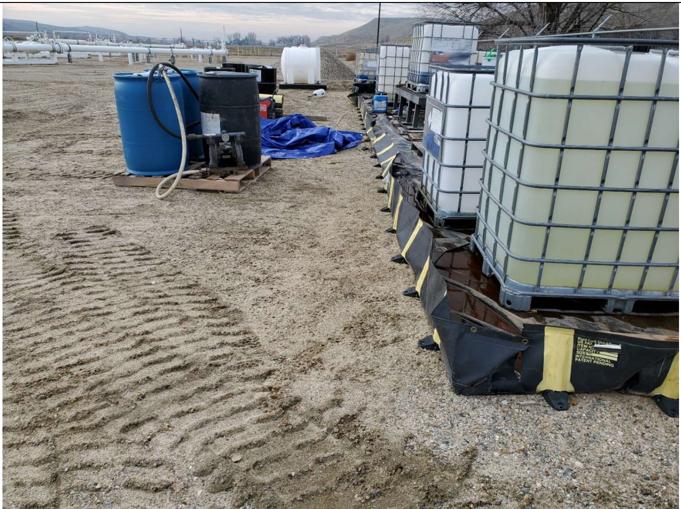
Secondary spill containment mat at west side of facility with corner tear, looking SW.
