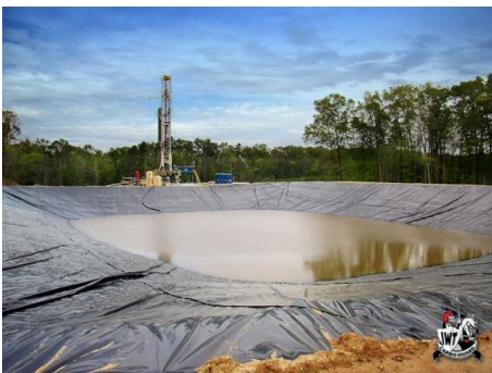
Figure 4-6 Lined pit designed to hold fluids during well drilling and completion - Source, IWT/ Cargo-Guard
