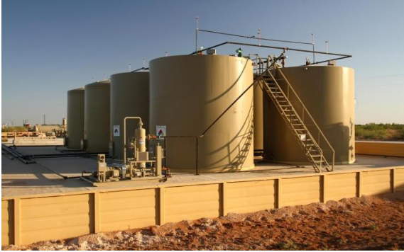
Figure 4-19 Secondary containment structure- Source, ©2014 Falcon Technologies and Services, Inc. All rights reserved.
