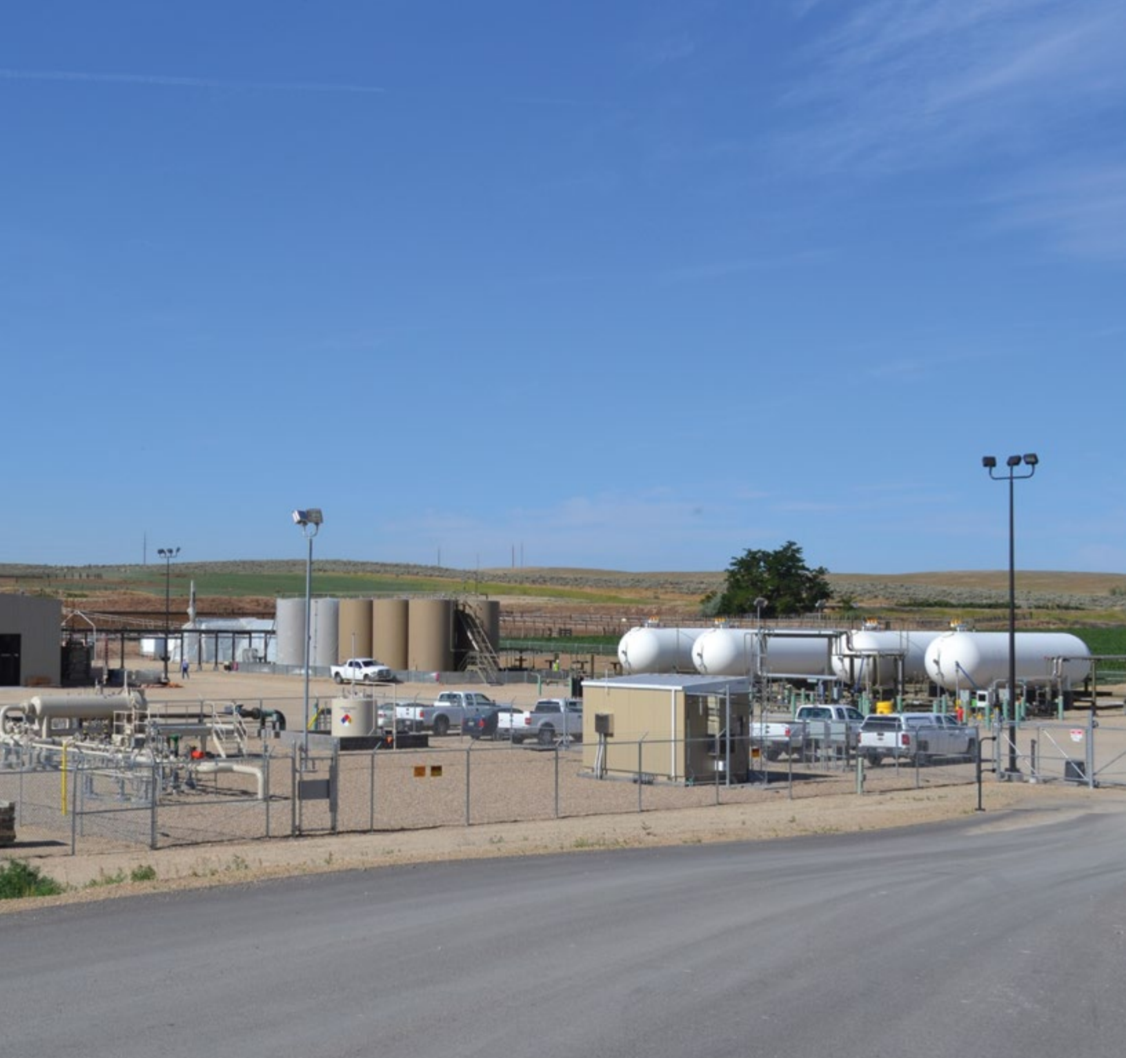
Highway 30 processing facility located in Payette County.
