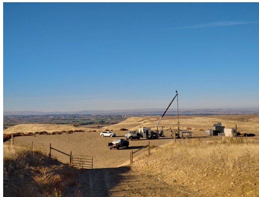
Kauffman #1-9 commencement of workover operations, October 2023.
