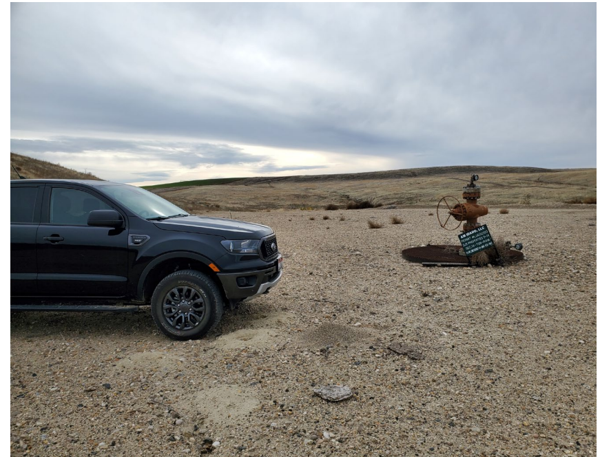
DJS Properties #2-14 wellhead during November 2023 field inspection. EPA permit number ID-2D001-A issued December 19, 2022 for Class II injection operations.
